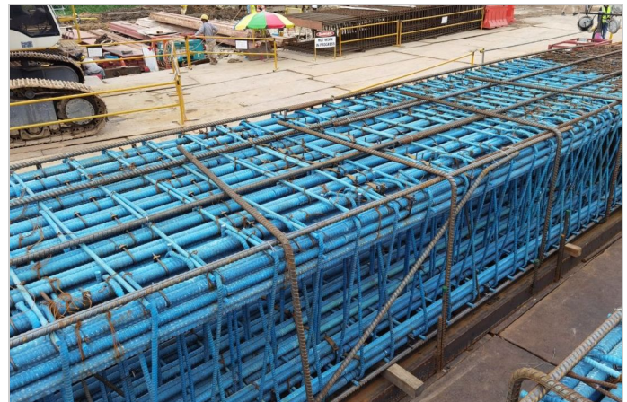
GFRP Soft Eye Reinforcement
