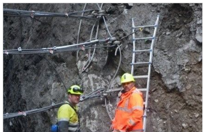
Longitudinal cable installation
