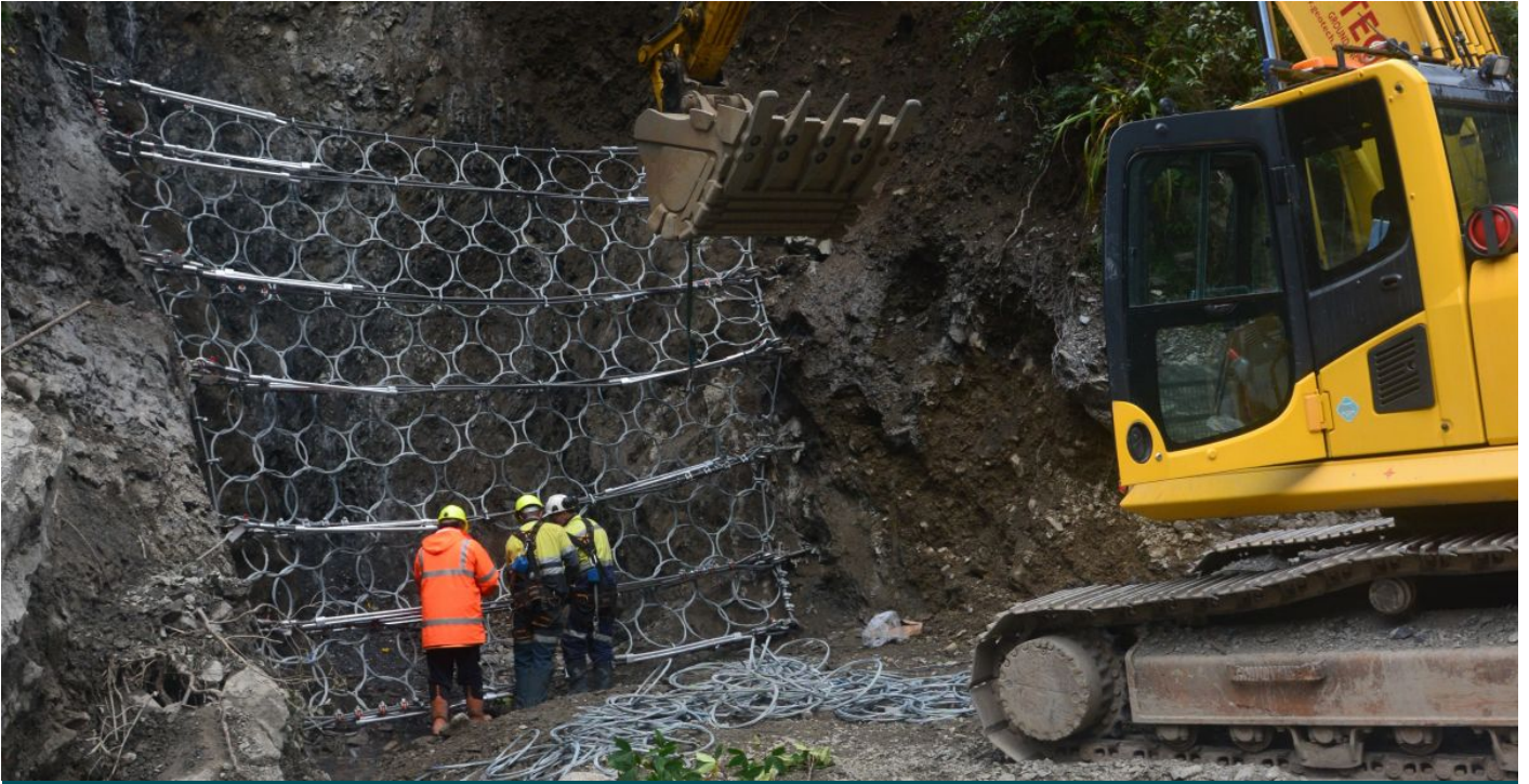
Debris flow fence nearing completion
