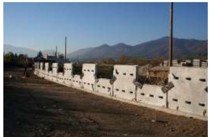
Start of construction:
