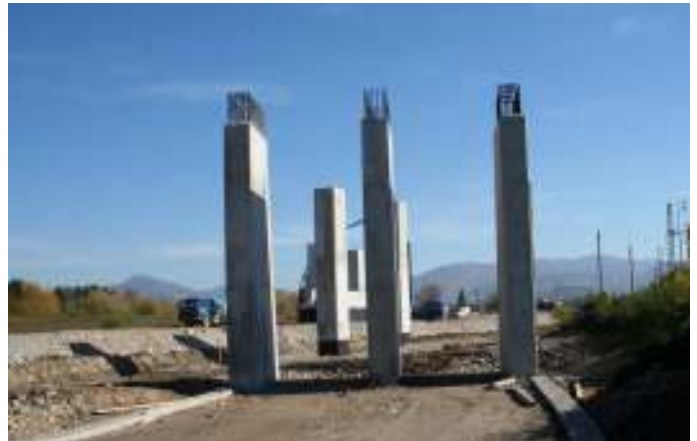
Start of construction:
