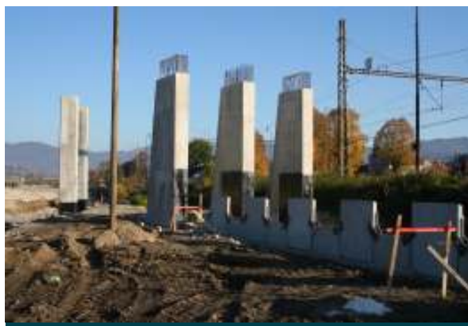
Start of construction
