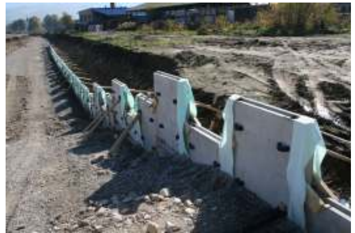
Start of construction
