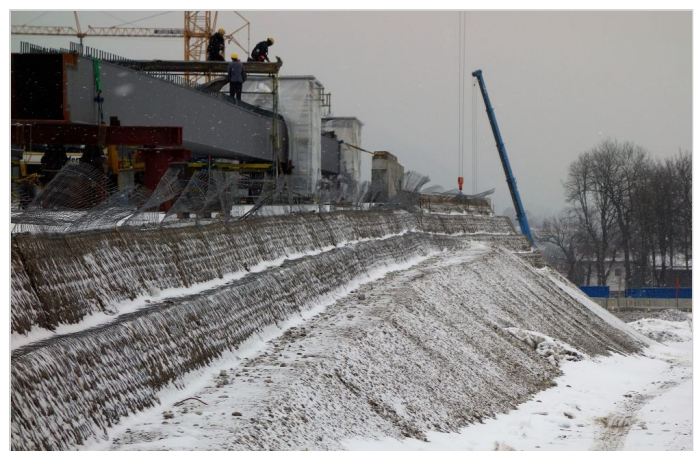
Construction phase: bridge decks on the terramesh wall
