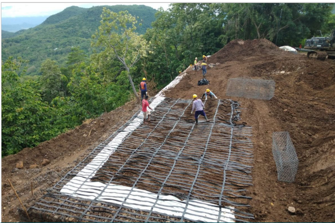
Paramesh Wall Installation
