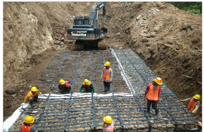
Paramesh Wall Installation
