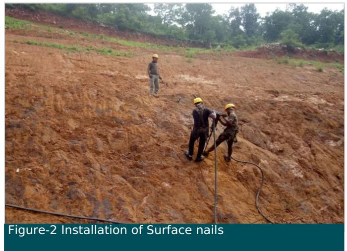
Figure-2 Installation of Surface nails
