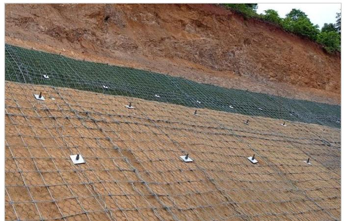
Figure-6 Overall site after the installation of slope protection system
