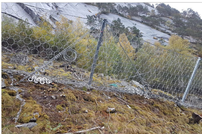
Share post / intermediate anchoring
