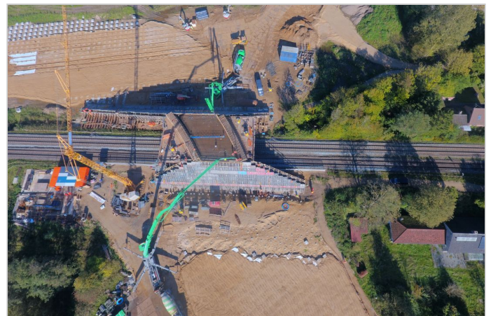
Drone aerial view after the covering of the pile caps
