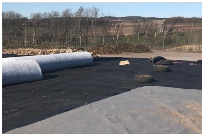
Construction phase: laying of the MacDrain W rolls
