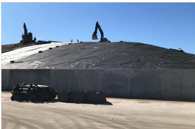
During the installation: capping detail
