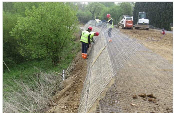
Construction phase: installation of Terramesh units
