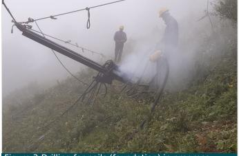
Figure 3-Drilling for nails (foundation) in progress
