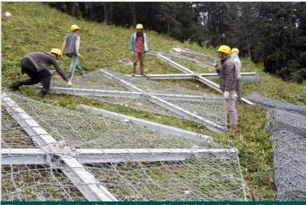
Figure 2- Onsite fabrication of individual Snow ErdoX
