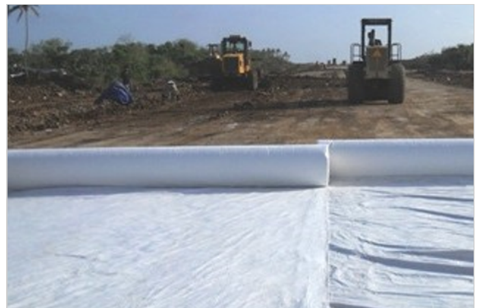
February 2011 - During Construction - Laying of Non-woven Geotextile
