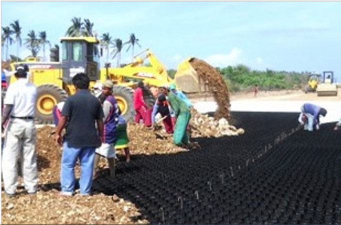
February 2011 - During Construction - Filling the MacCells
