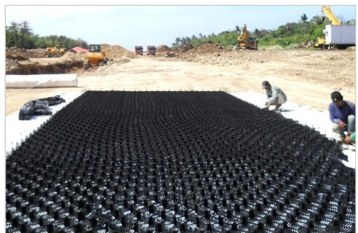
February 2011 - During Construction - Laying and Expanding of MacCell
