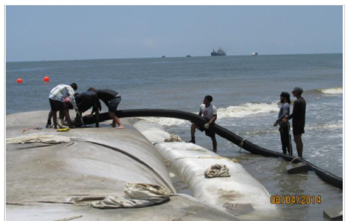
Photo 2: During construction of groyne bund
