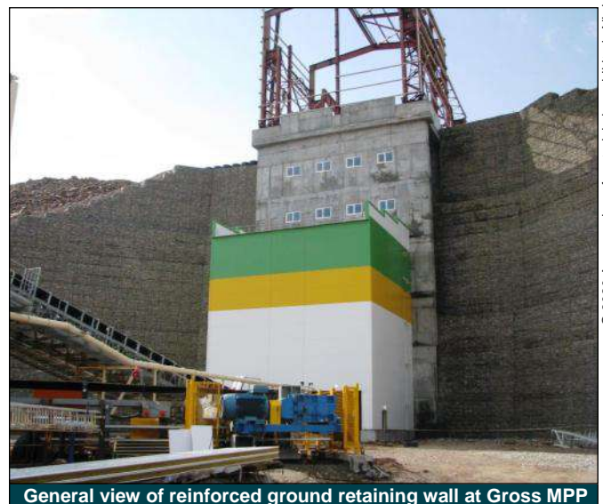
General view of reinforced ground retaining wall at Gross MPP
