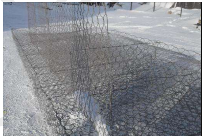
Assembly of gabion structures on site
