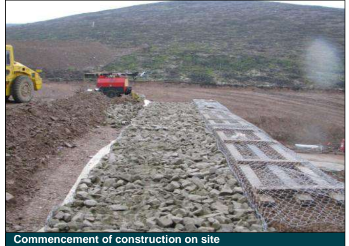
Commencement of construction on site
