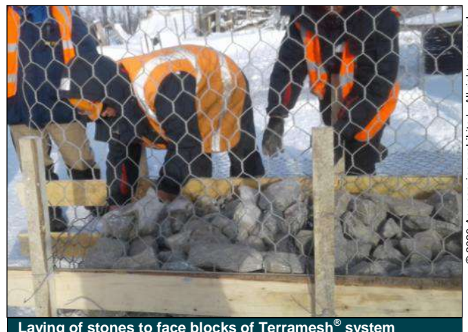
Laying of stones to face blocks of Terramesh® system
