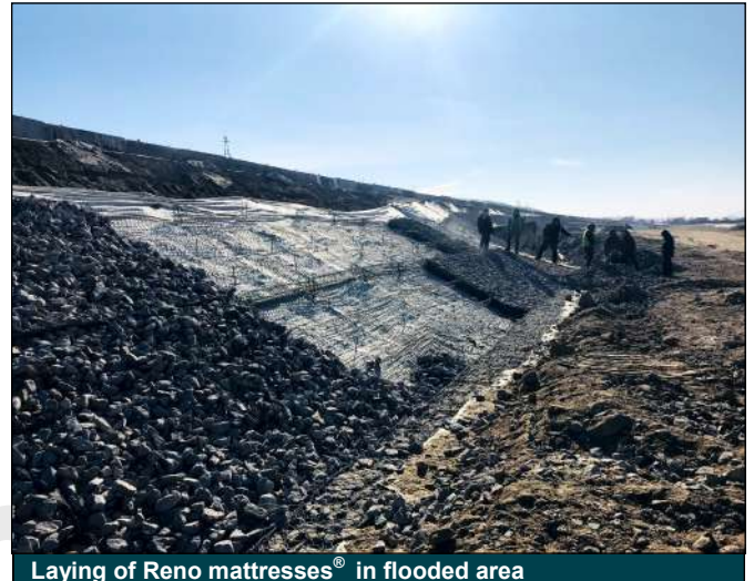
Laying of Reno mattresses ® in flooded area
