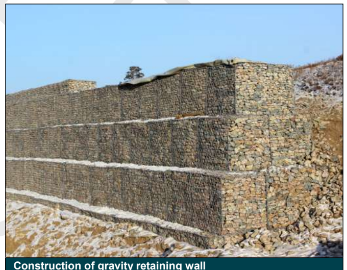
Construction of gravity retaining wall
