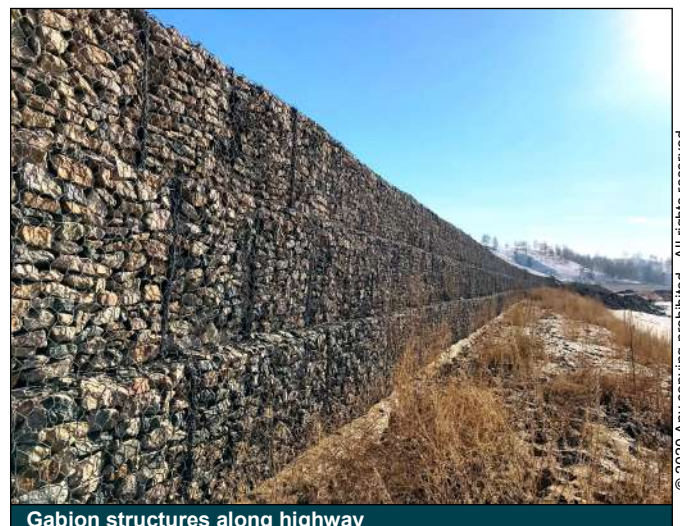
Gabion structures along highway
