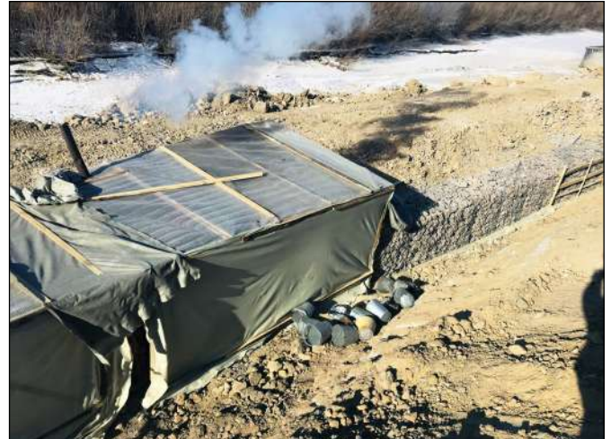
Mobile heated shed for gabion structures
