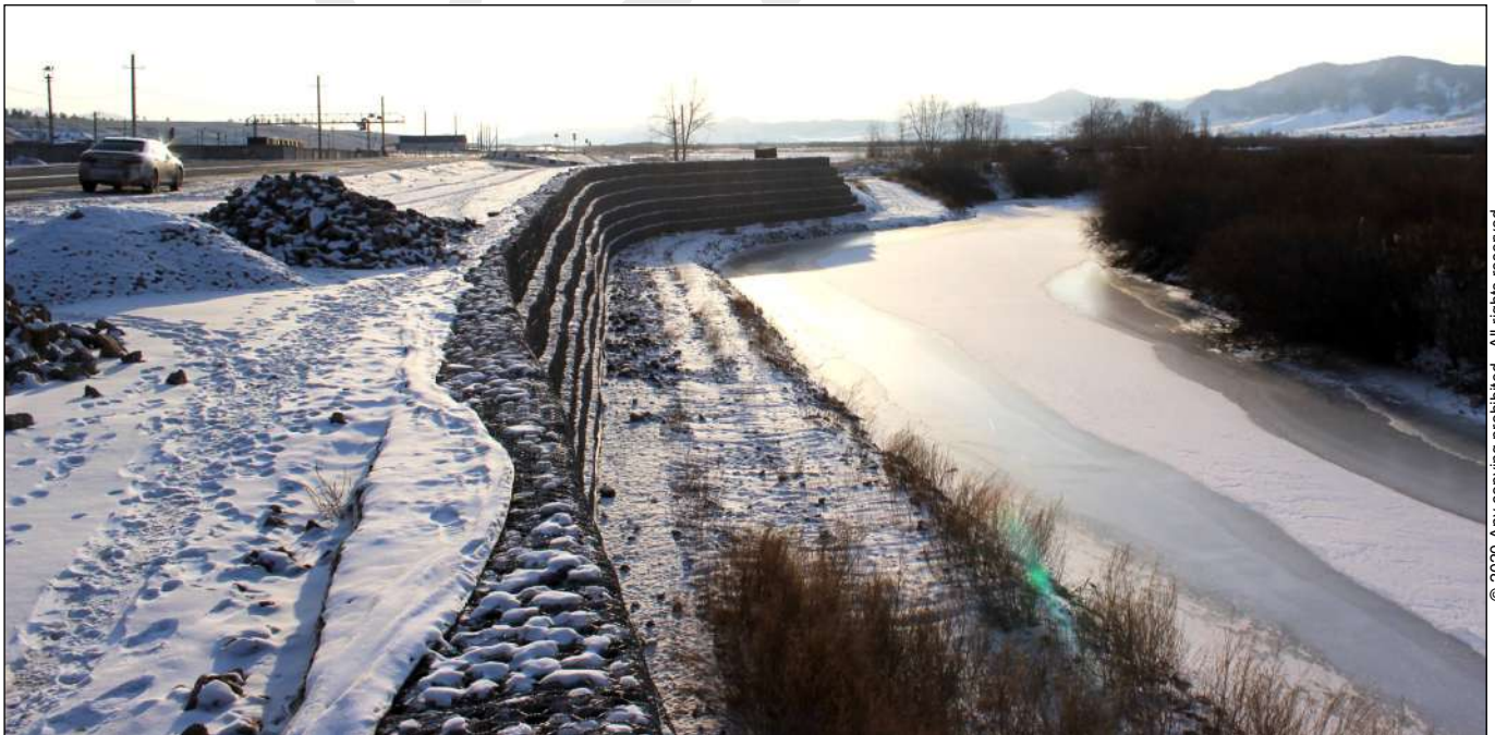
Completed Terramesh® reinforced ground system along Selenga river
