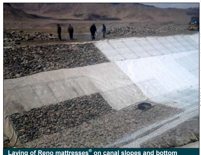
Laying of Reno mattresses® on canal slopes and bottom
