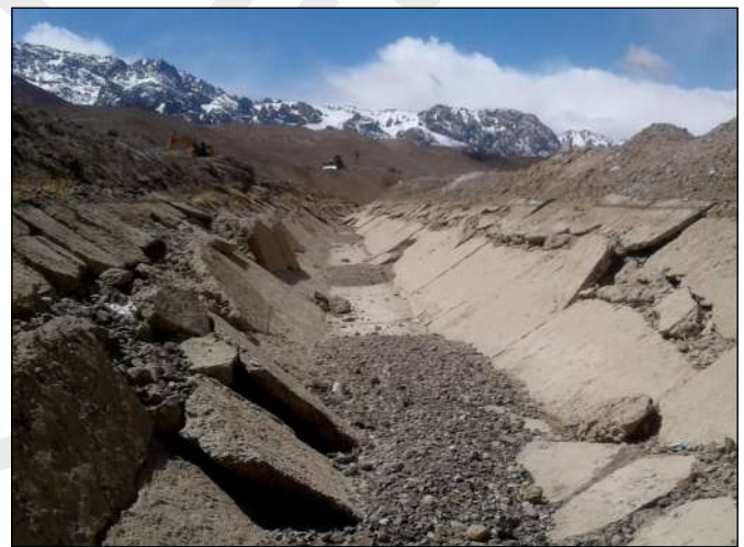
River diversion canal of Aksu HPP before reconstruction
