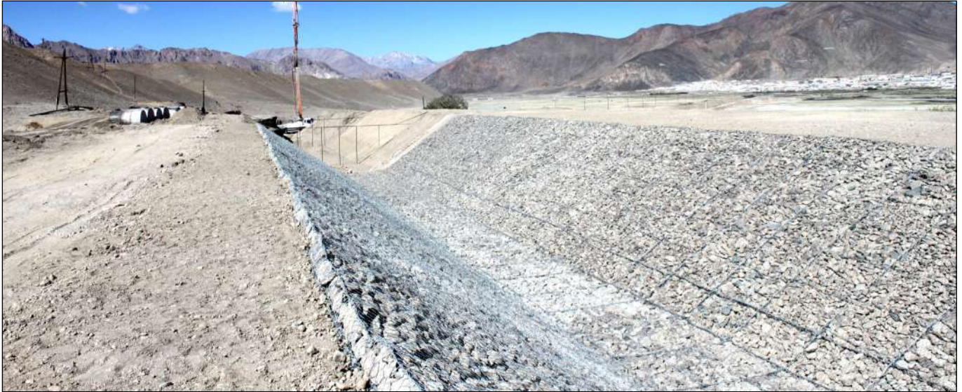
Diversion canal of Aksu HPP reinforced with Reno mattresses®
