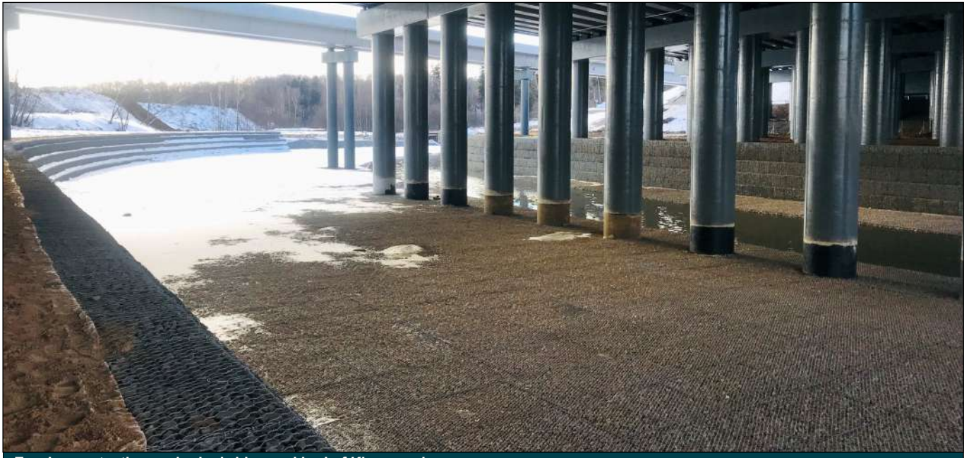
Erosion protection under the bridge and bed of Klyazma river
