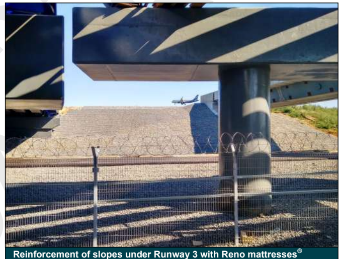
Reinforcement of slopes under Runway 3 with Reno mattresses ®
