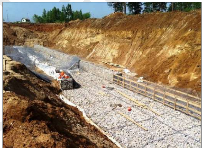
River bed reinforcement with Reno mattresses ®
