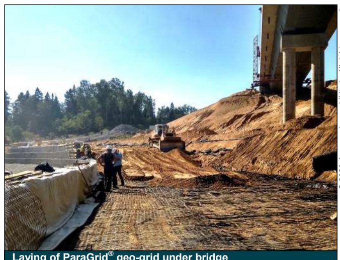
Laying of ParaGrid ® geo-grid under bridge
