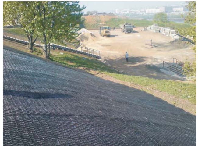
Pic.4 During construction
