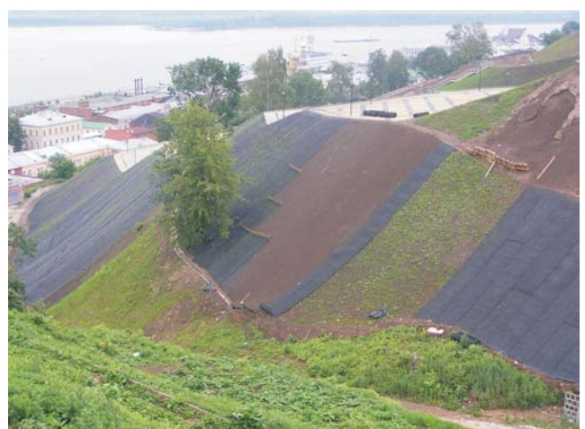
Pic.5 During construction
