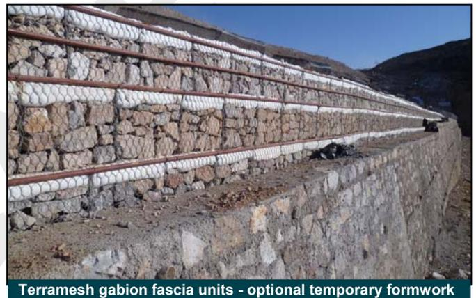
Terramesh gabion fascia units - optional temporary formwork
