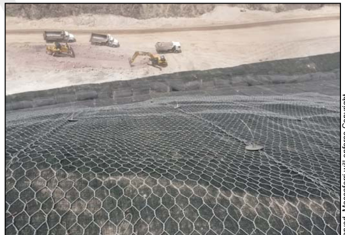
After construction and awaiting vegetation establishment
