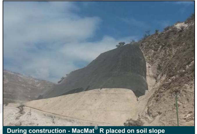
During construction - MacMat® R placed on soil slope
