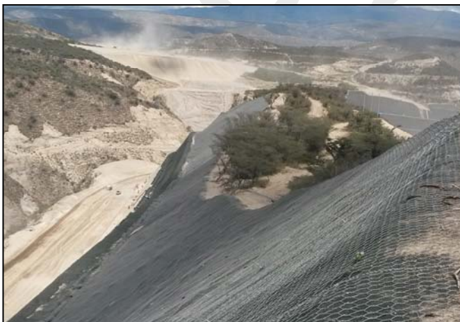
After construction and awaiting vegetation establishment
