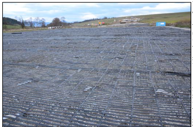
ParaLink® in place ready to receive embankment construction
