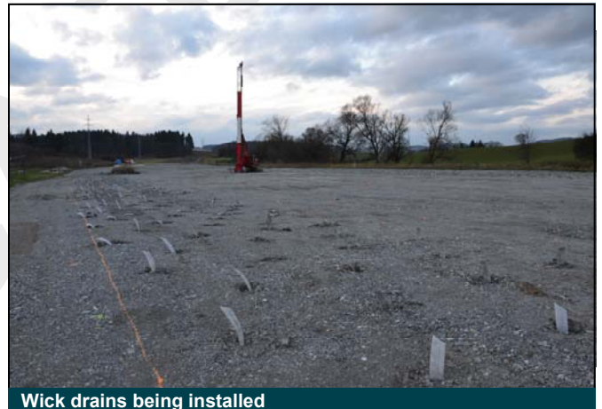
Wick drains being installed
