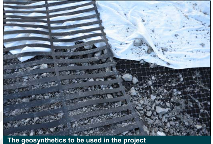
The geosynthetics to be used in the project
