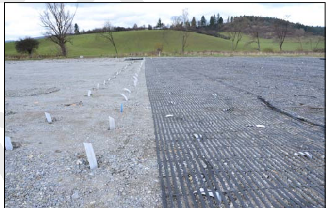
Laying of ParaLink® - note vertical wick drains in place
