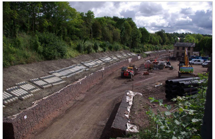
Retaining structure being installed at Gorebridge Station
