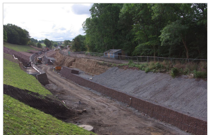
Area of Ladybray, installing the Gabion retaining structure
