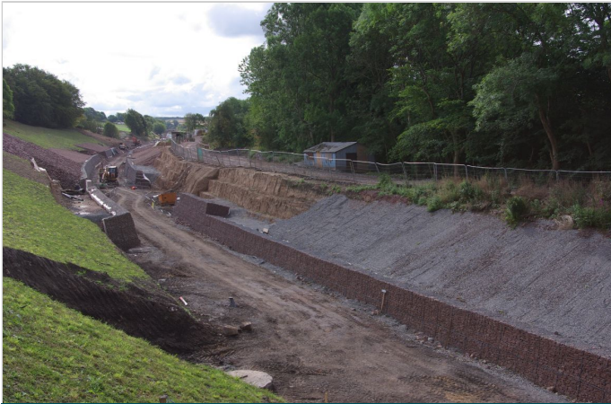
Area of Ladybray with Gabion retaining wall installed
