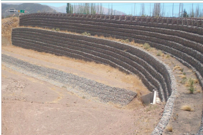
Toe scour protection with Reno Mattresses
