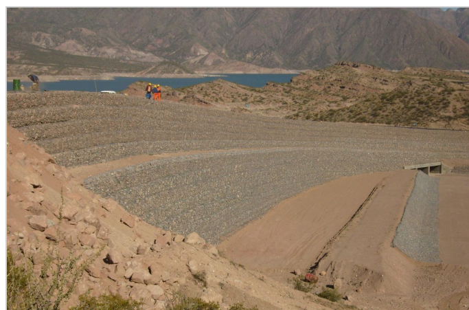
Retaining wall with TerraMesh System
