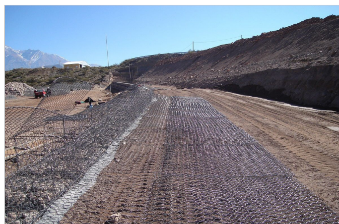
TerraMesh System - installation details
