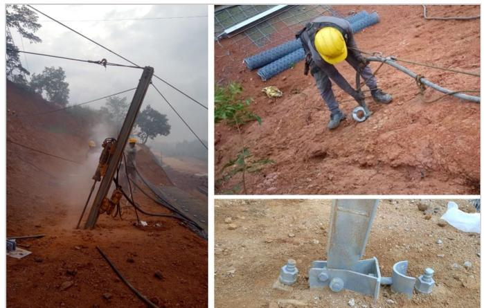
Figure-2 Activities related to installation of barrier posts
