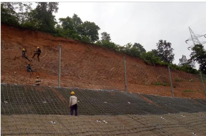
Figure-5 Installation of primary and secondary mesh (MacRing + DT mesh)
