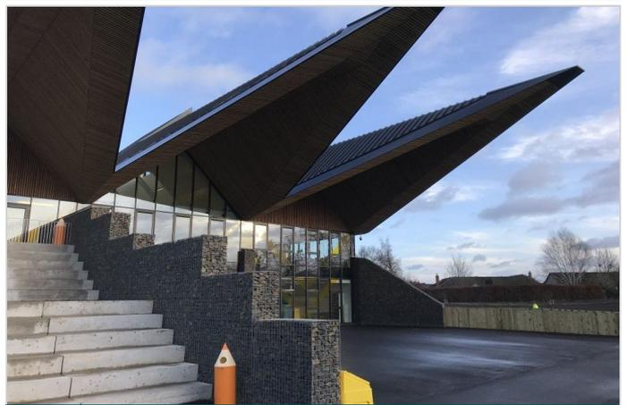
Free standing gabion wall with iconic roof design
