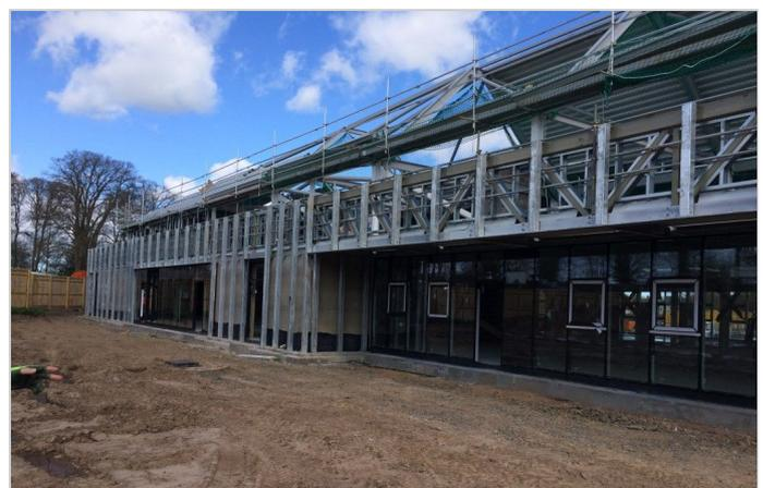
Steel sections used to support gabion cladding
