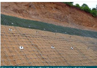
Figure-6 Overall site after the installation of slope protection system
