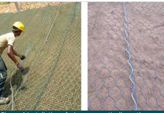
Figure-4 Installation of wire rope vertically on the edges of DT mesh
