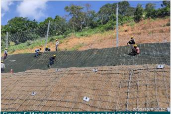
Figure-5 Mesh installation over nailed slope face
