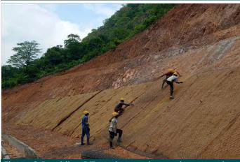
Figure-3 Providing DT mesh over the erosion control
