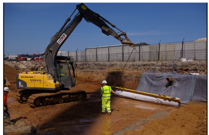
MacLine® during installation
