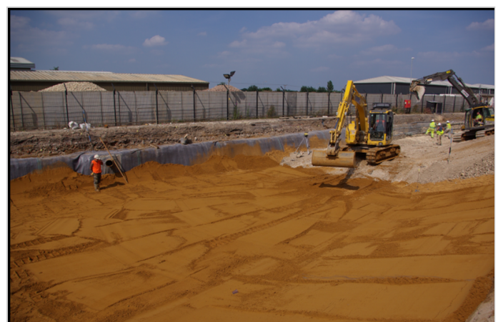
MacLine® and Gabion installation
