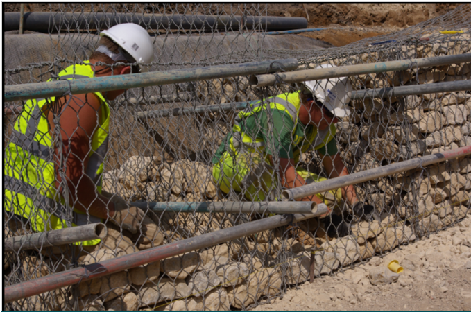
Installation of double twist gabions
