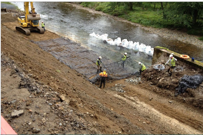
Structural backfill laid onto the reinforcement grids—ParaGrid
