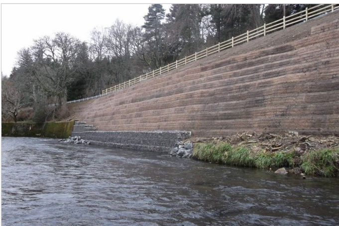
Completed Green Terramesh® slope stabilisation with the Terramesh system
