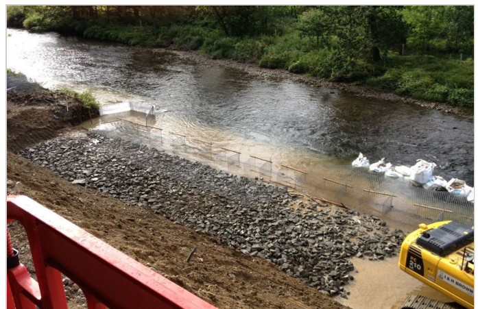
Excavated ground then laid with locally sourced rock
