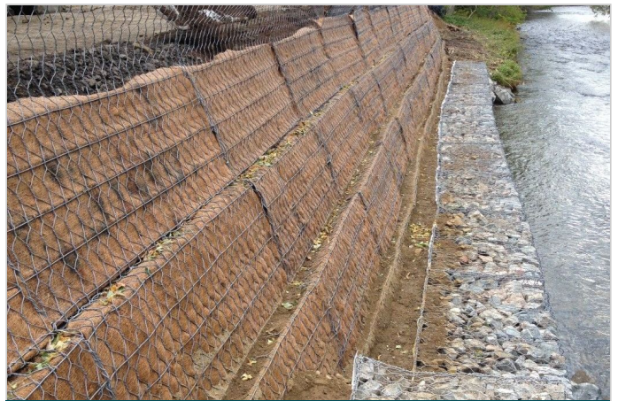
Locally sourced gabion fill at the bottom of the river.
