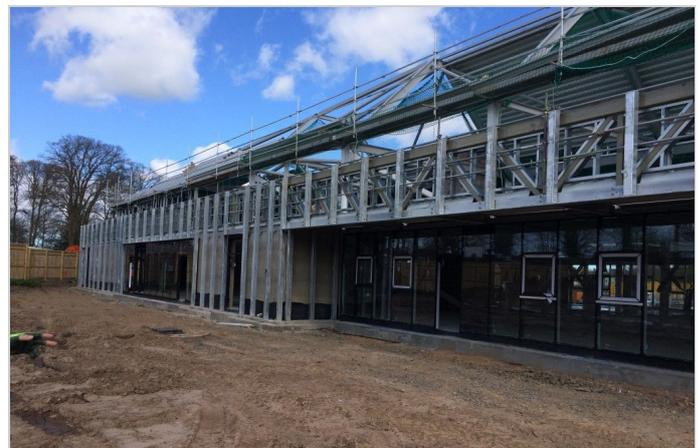
Steel sections used to support gabion cladding
