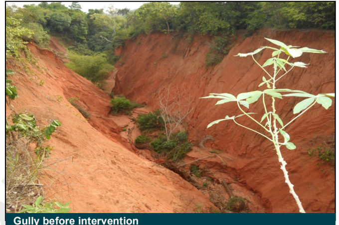
Gully before intervention
