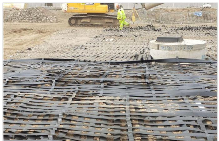
Layers of ParaLink® can be installed perpendicular to increase protection
