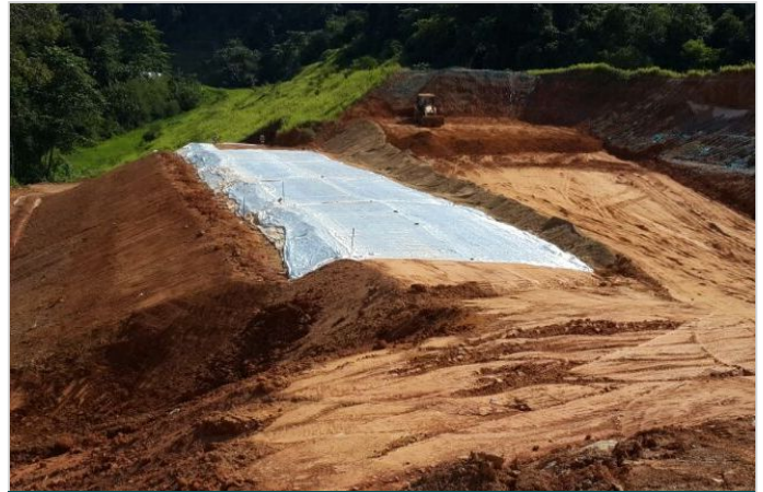
Woven Geotextiles used as reinforcements for the road widening
