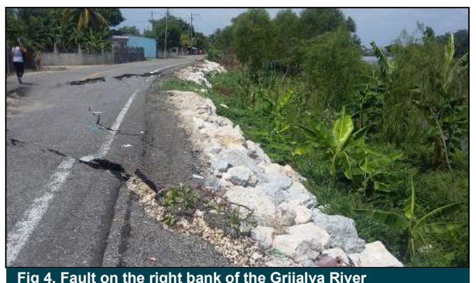
Fig 4. Fault on the right bank of the Grijalva River
