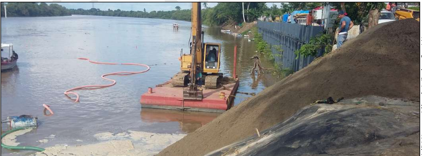
Fig 6. Site ready for material placement
