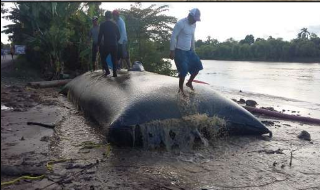
Fig 8. Filled and drained process MacTube®
