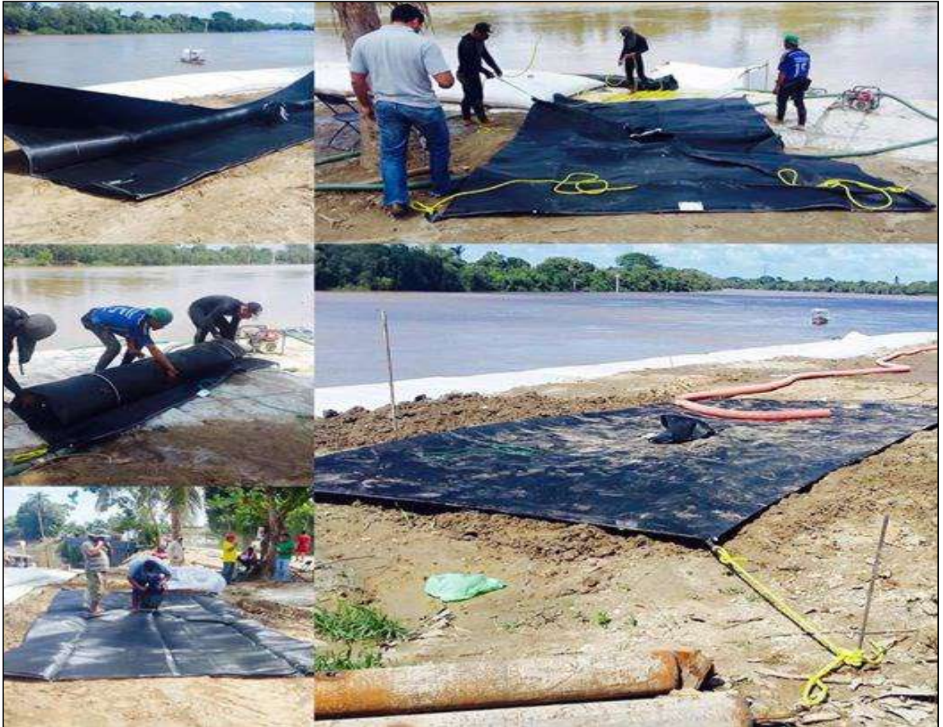
Fig 5. Preparation site for MacTube® W17.10 before being filled
