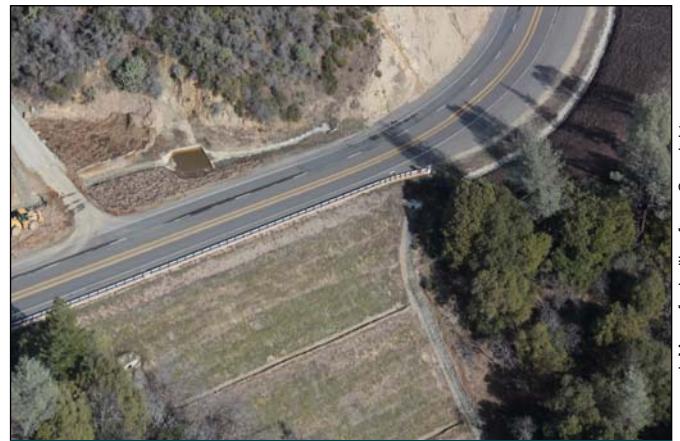
Completed project with collectors and benches installed
