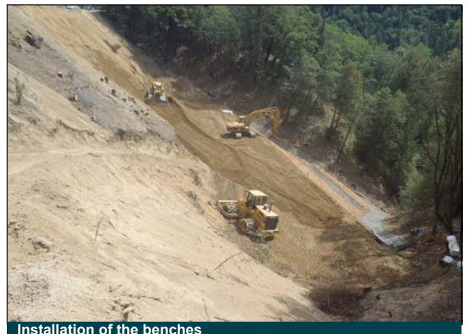
Installation of the benches
