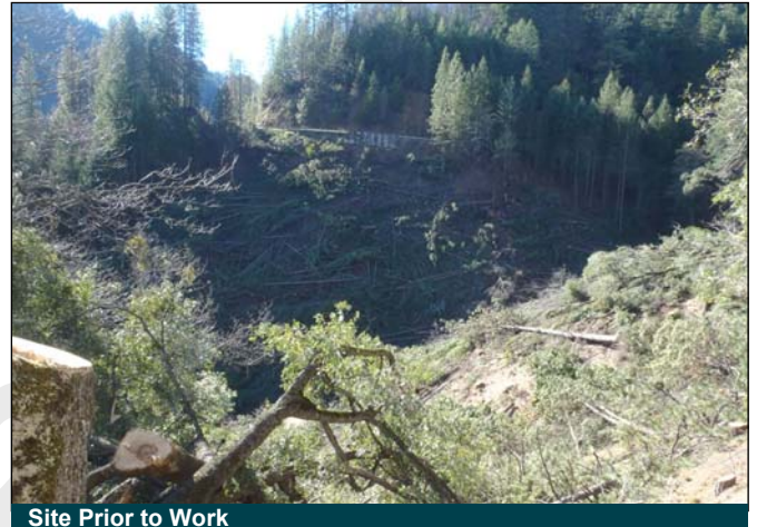
Site Prior to Work
