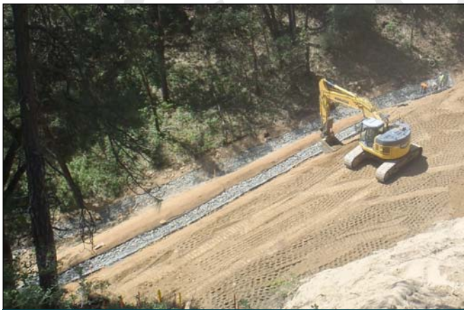
Installation of the Gabion mats on the benches
