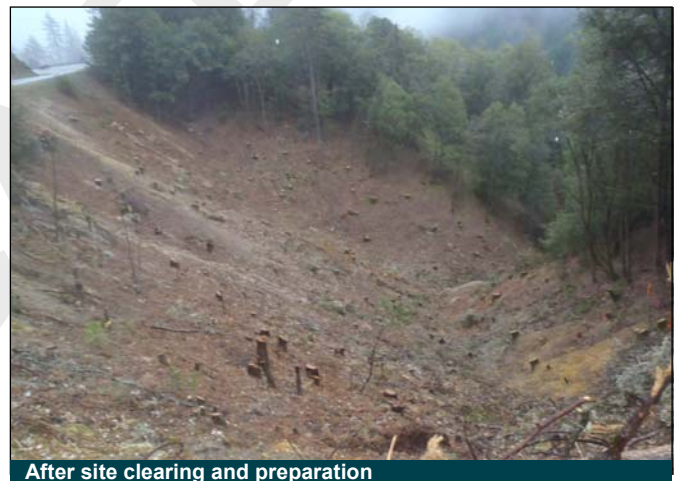
After site clearing and preparation
