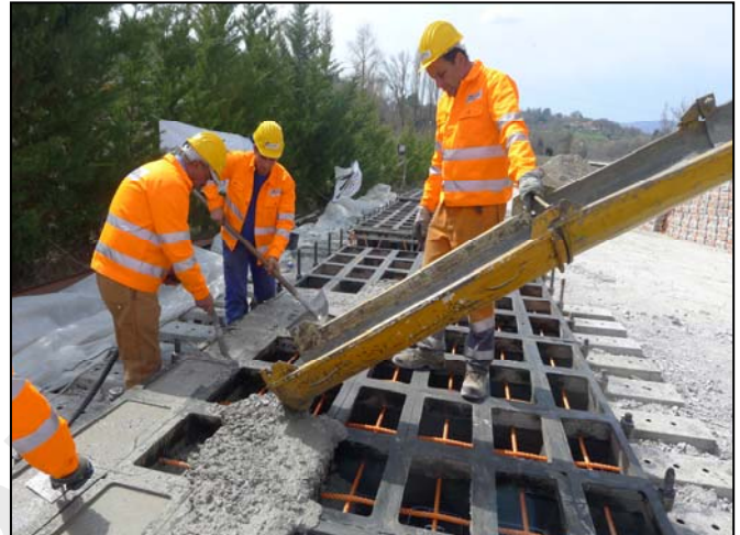
ACBM mattresses casting operations
