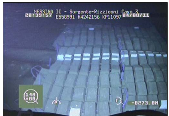
Installed ACBM Mattresses
