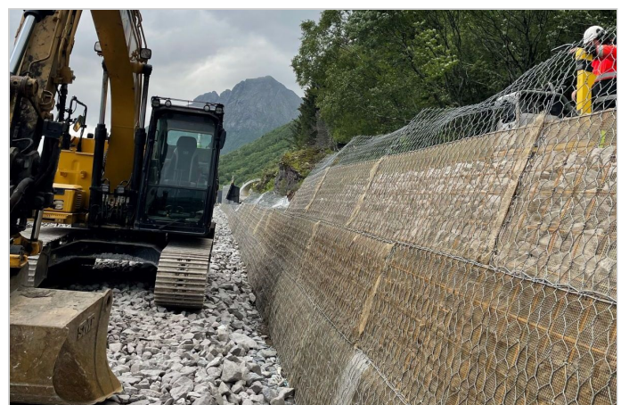
During the installation of GTM DUO units
