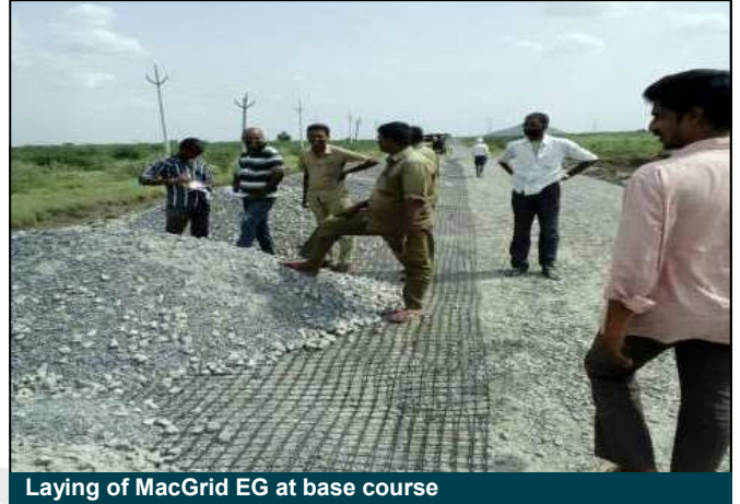
Laying of MacGrid EG at base course
