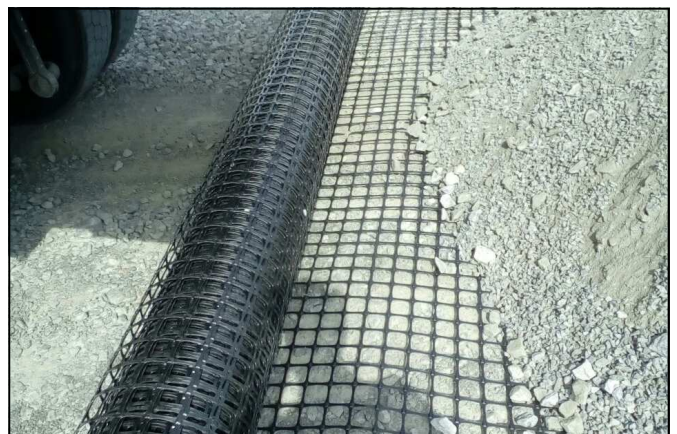
Unrolling & laying of MacGrid EG at base course (WMM)
