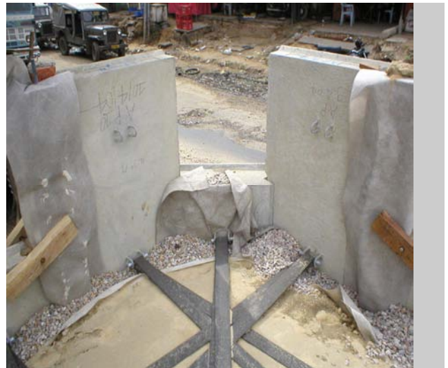
Fig 9,10. Laying of Paraweb at the corners
