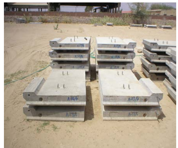
Fig 3. Concreted Panels ready for construction
