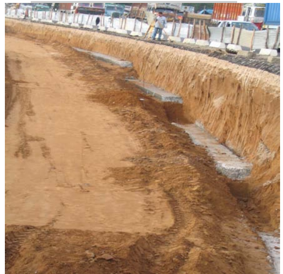
Fig 1. Construction of levelling pad
