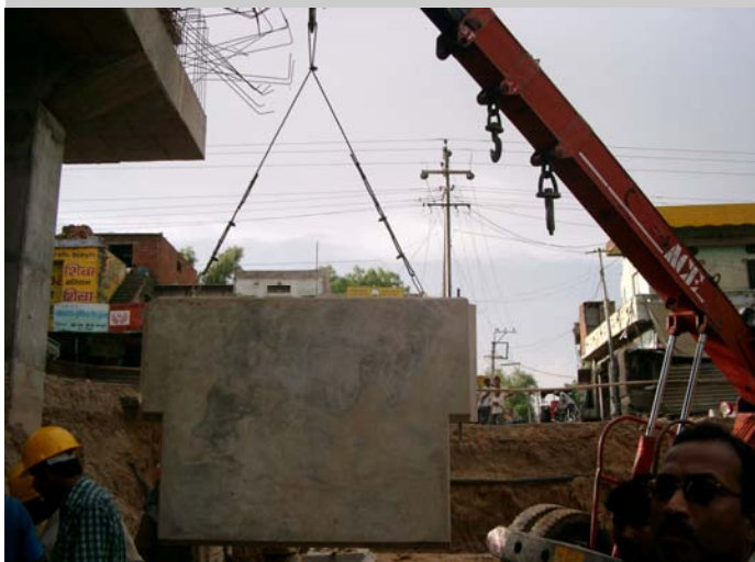
Fig 4,5.Erection & laying of facia Panels
