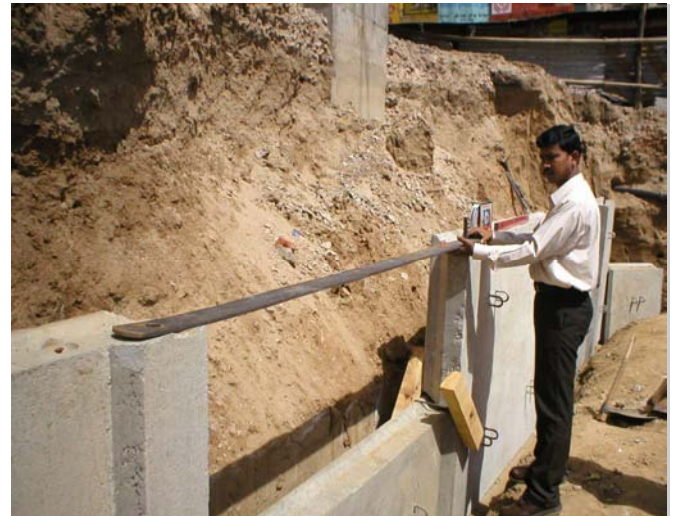
Fig 4,5.Erection & laying of facia Panels
