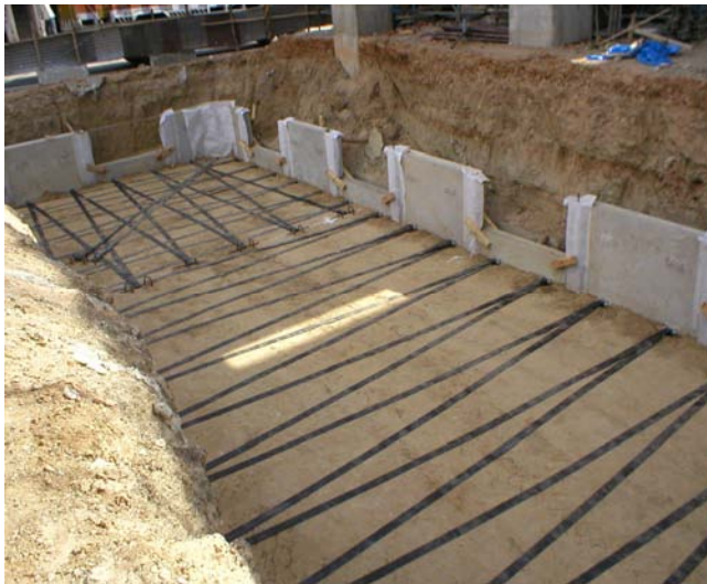
Fig 9,10. Laying of Paraweb at the corners
