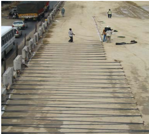
Fig 7. Laying of Paraweb
