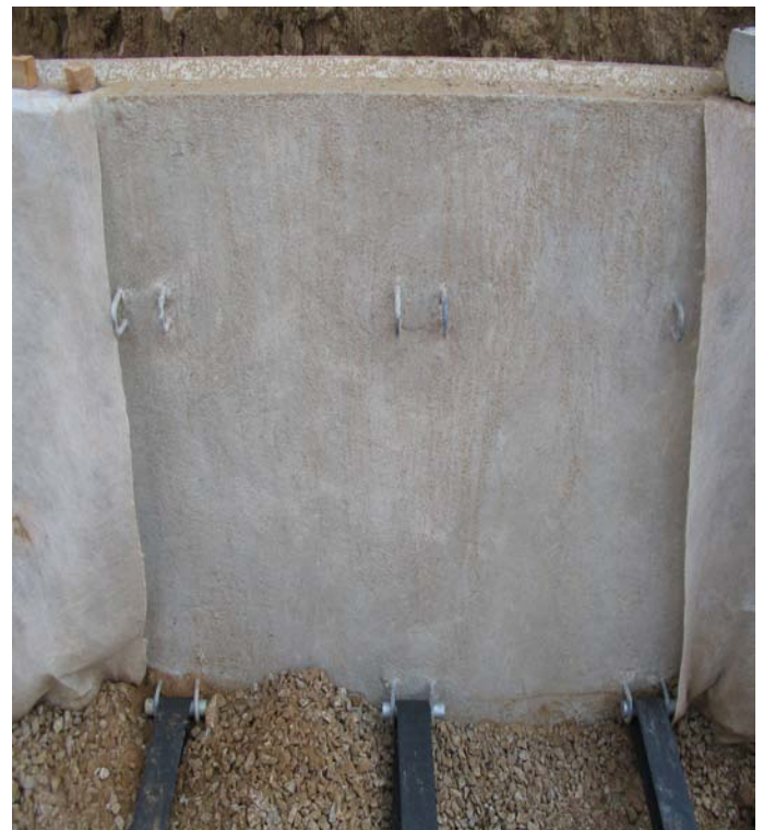
Fig 6.Connection between facia panel & Paraweb
