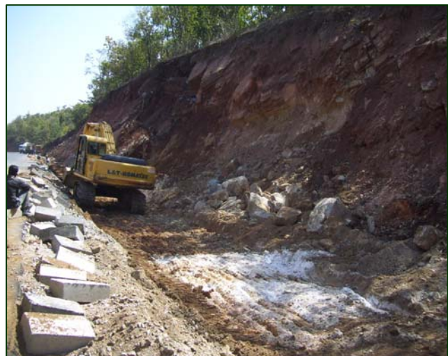
Photo 2: Site-Removal of excess earth
