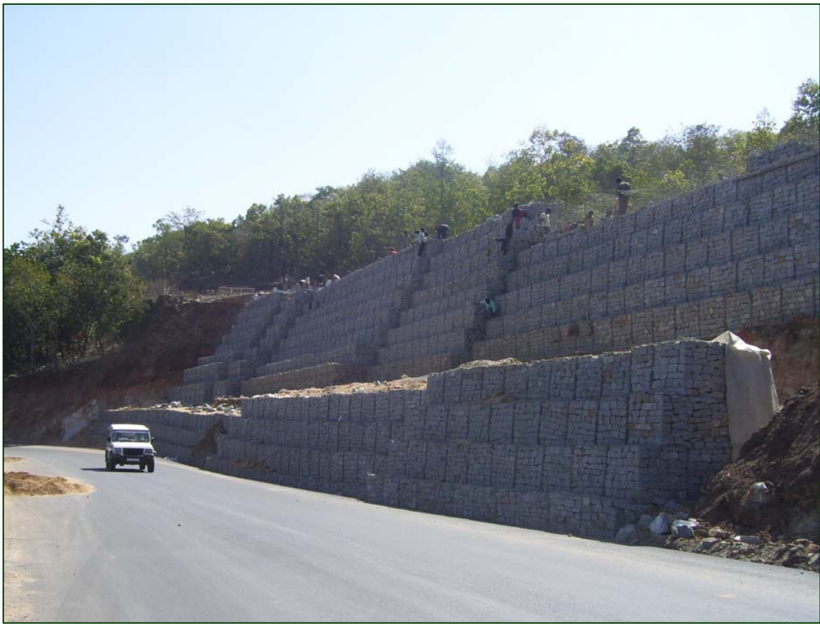
Photo 7: Completed Maccaferri Gabion Structure
