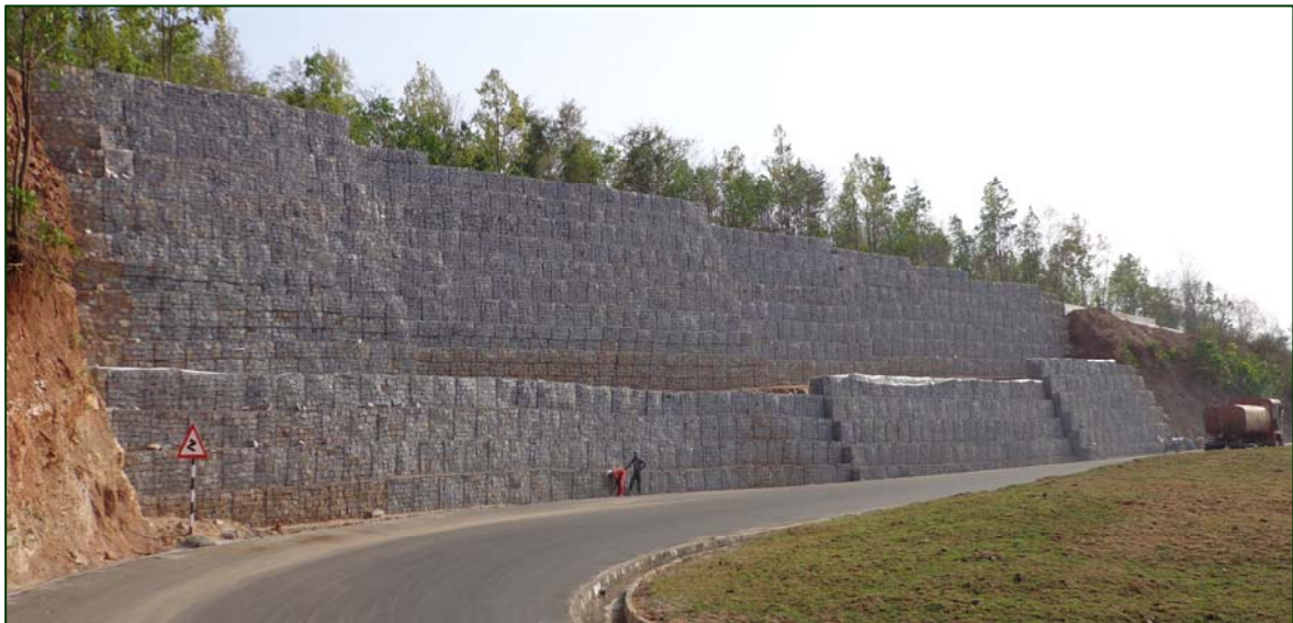
Photo 8: Completed Maccaferri Gabion Structure
