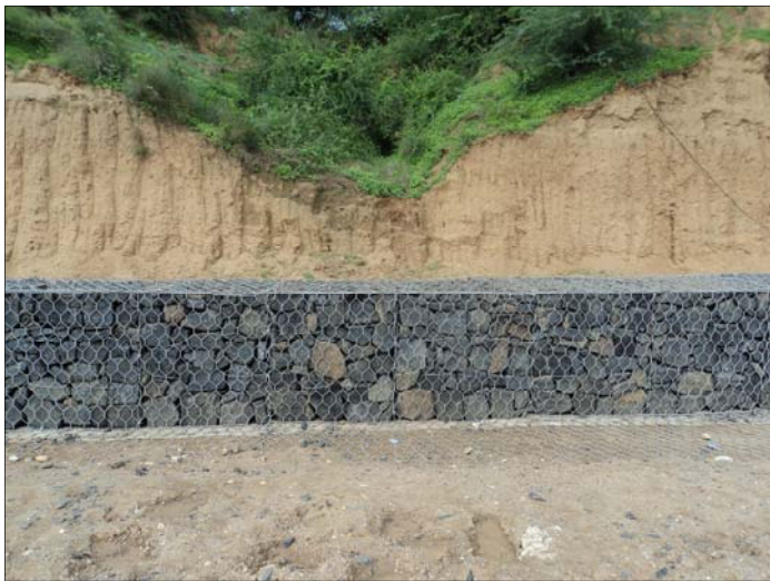
Photo 4 : During Construction - Gabion facia.
