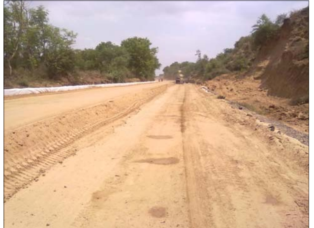
Photo 1 : Initial Stage of Construction
