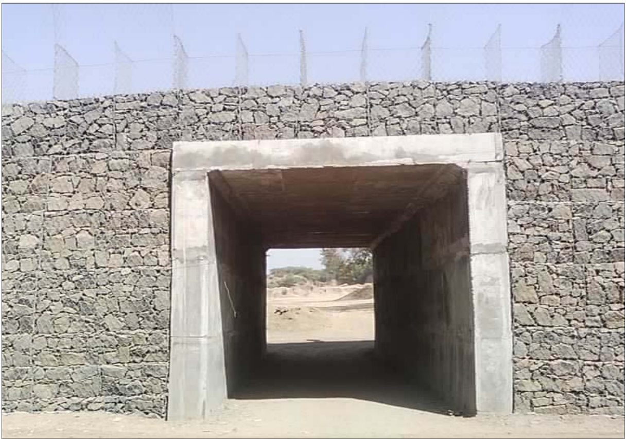
Photo 7 : Construction stage—Terramesh system with Box Culvert
