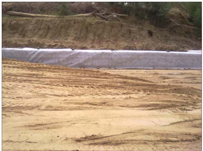
Photo 5 : Terramesh system wrapped with Geotextile
