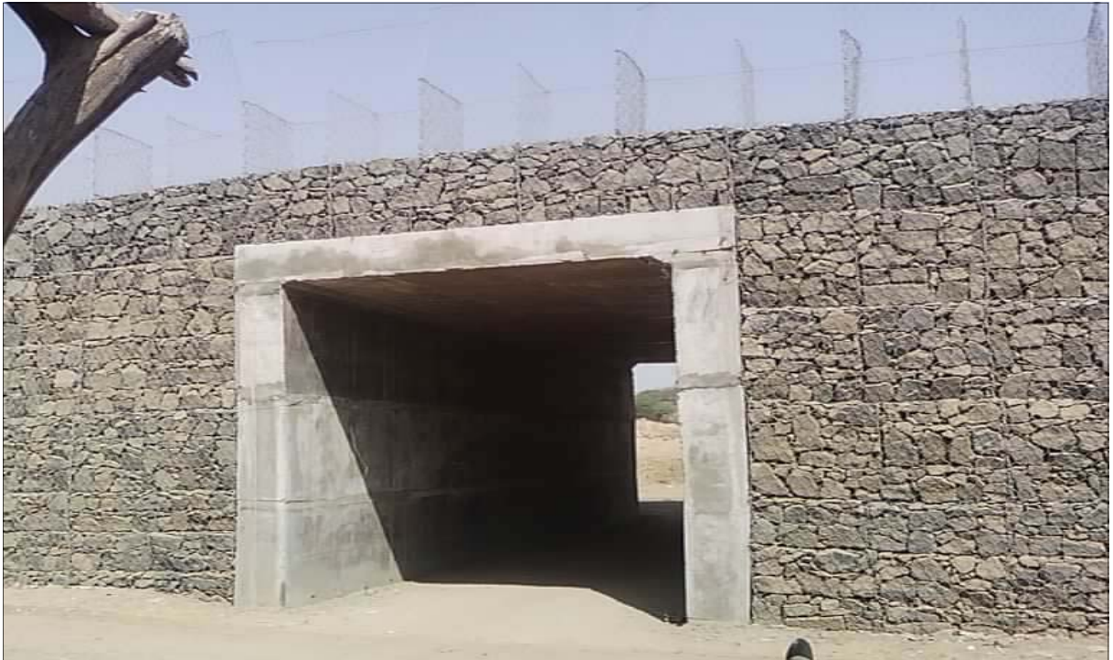
Photo 6 : Construction stage—Terramesh system with Box Culvert
