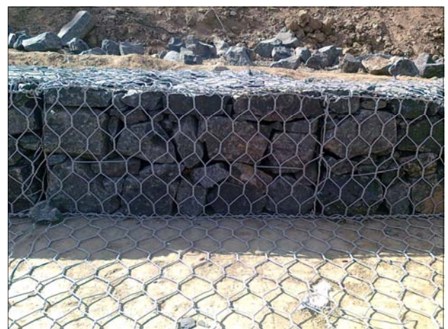
Photo 3 : During Construction - Gabion facia.
