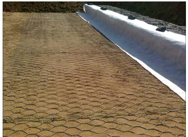
Photo 2 : Installation of Non woven Geotextile
