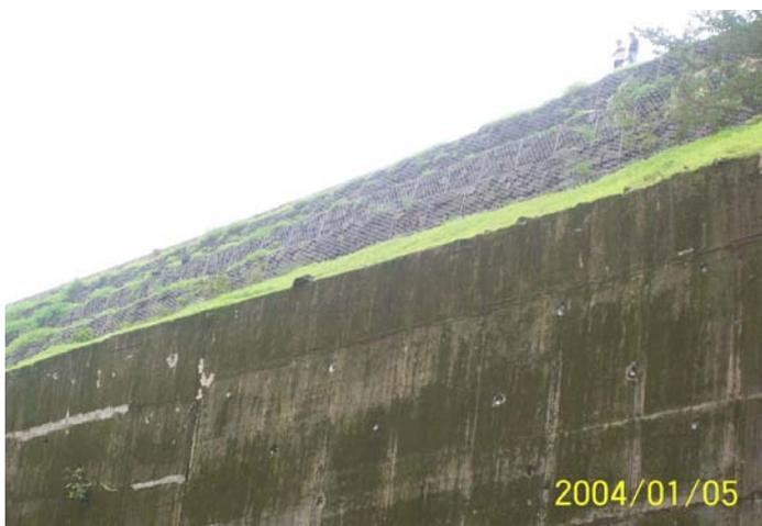
**Photo 8: Gabions on the valley side where global stability was critical**
