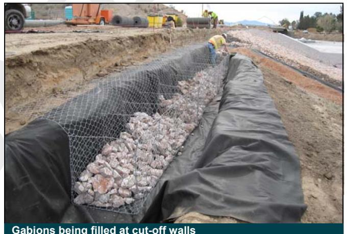
Gabions being filled at cut-off walls
