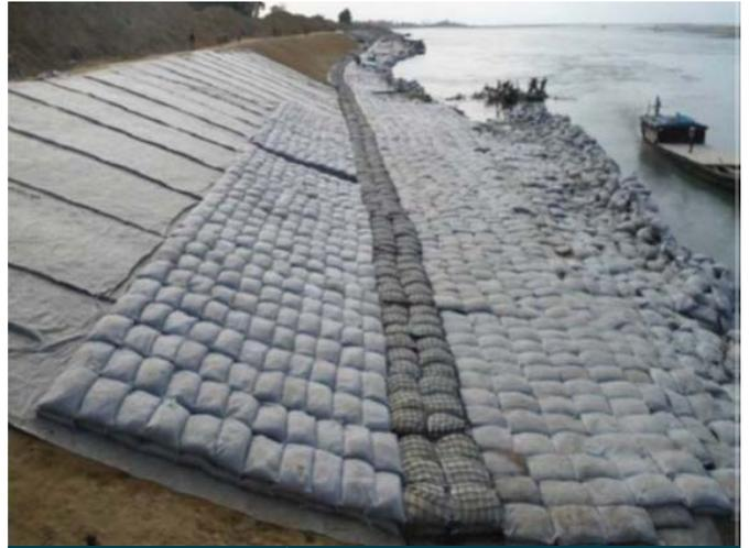
Placement of MacBags®. Note filter geotextile beneath units
