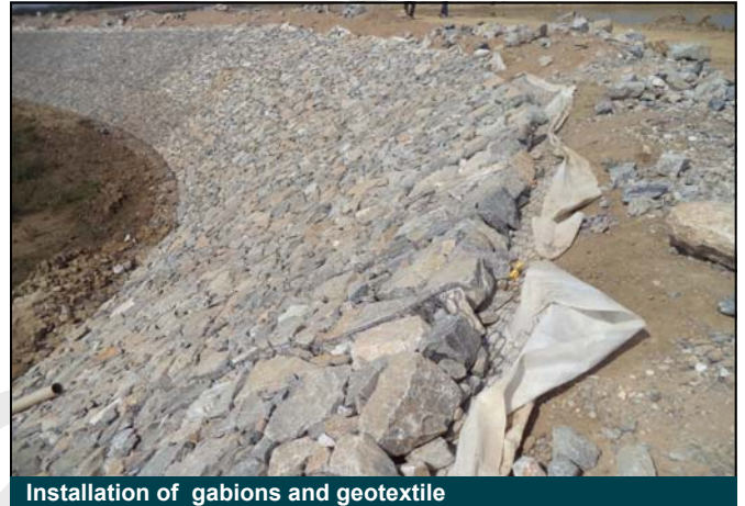
Installation of gabions and geotextile
