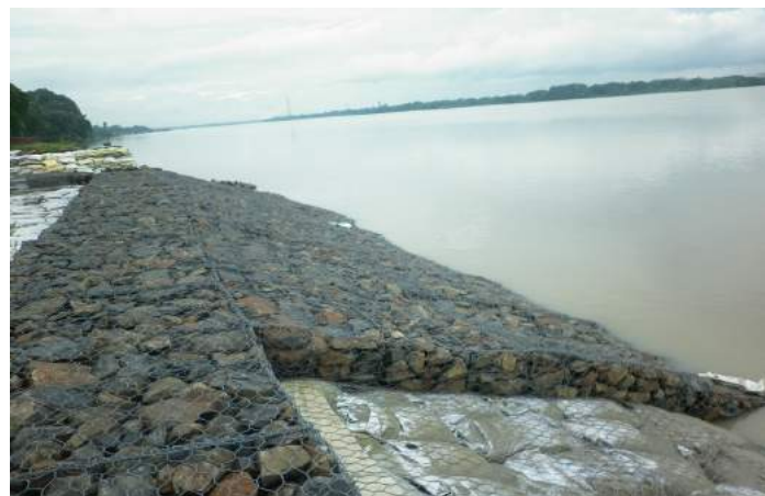
Photo 6 : Placement of the Gabion Mattress
