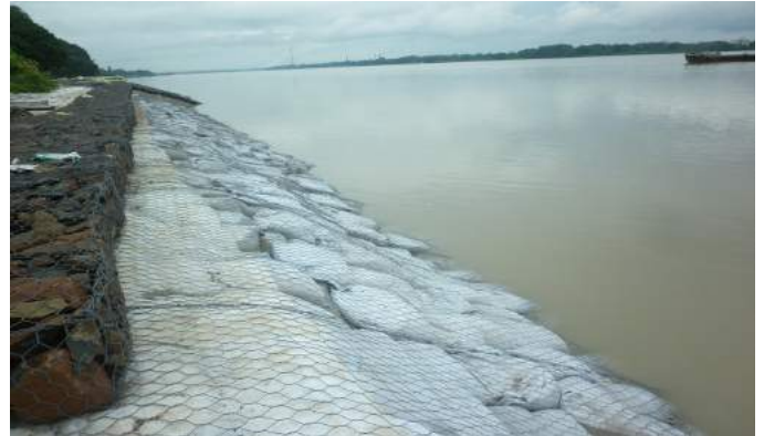
Photo 4 : Placed MacBags on the Slope
