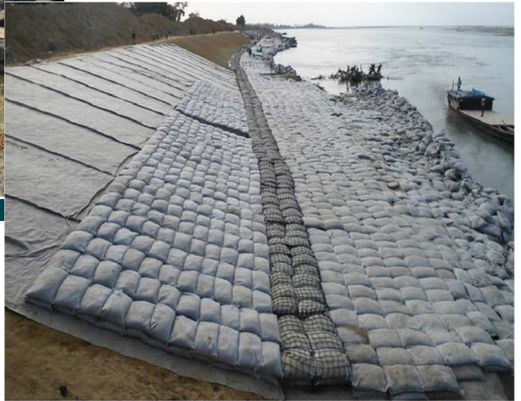
Photo 5 Placement of MacBags™ on the river bank
