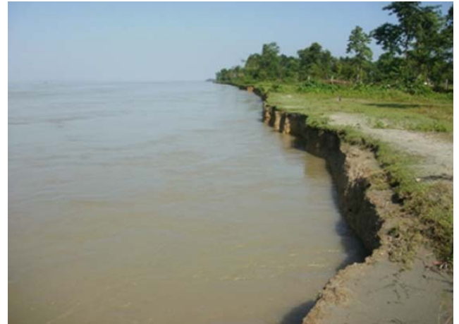
Photo 1 Scouring of the banks of Brahmaputra River
