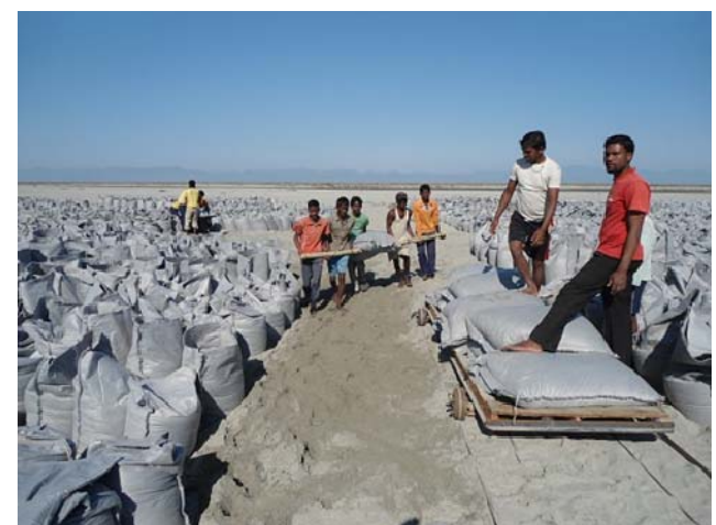
Photo 3 Filling & transportation of MacBags™
