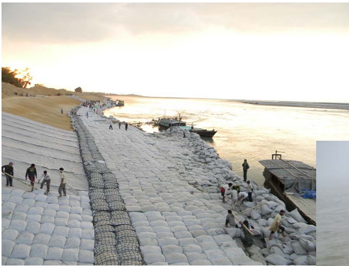
Photo 6 Placement of MacBags™ on the river bank
