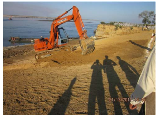
Photo 2 Dressing of slope
