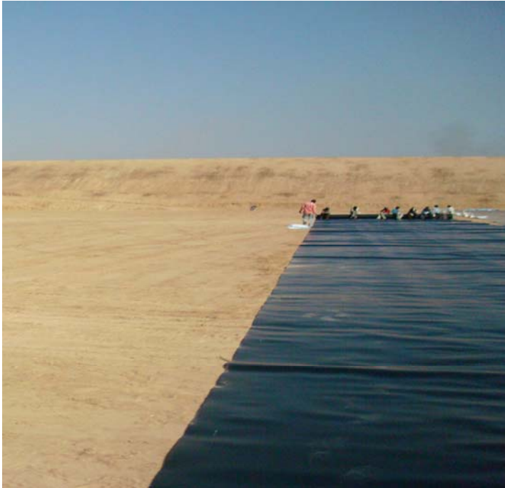
Photo 3,4. Unravelling the HDPE Membrane
