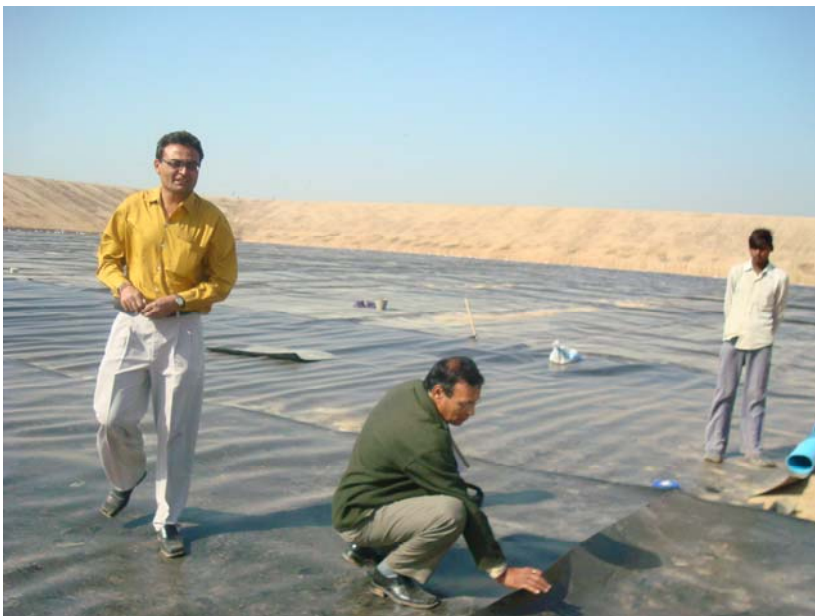
Photo 5. Preparation of the joints for stitching .
