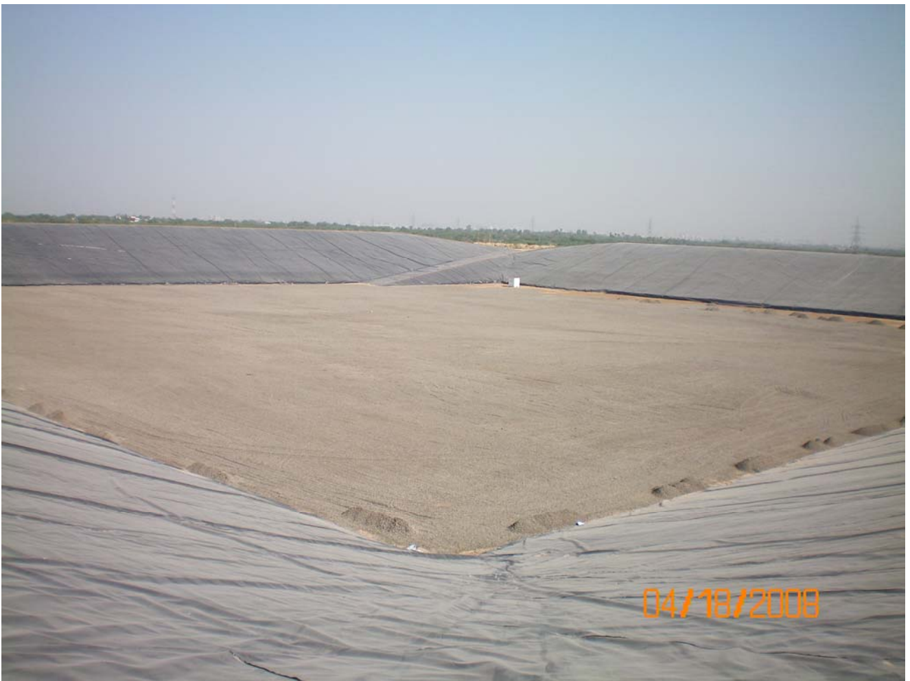
Photo 12. Base liner and side liner laying completed
