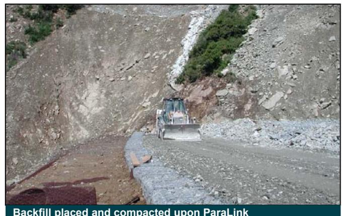
Backfill placed and compacted upon ParaLink
