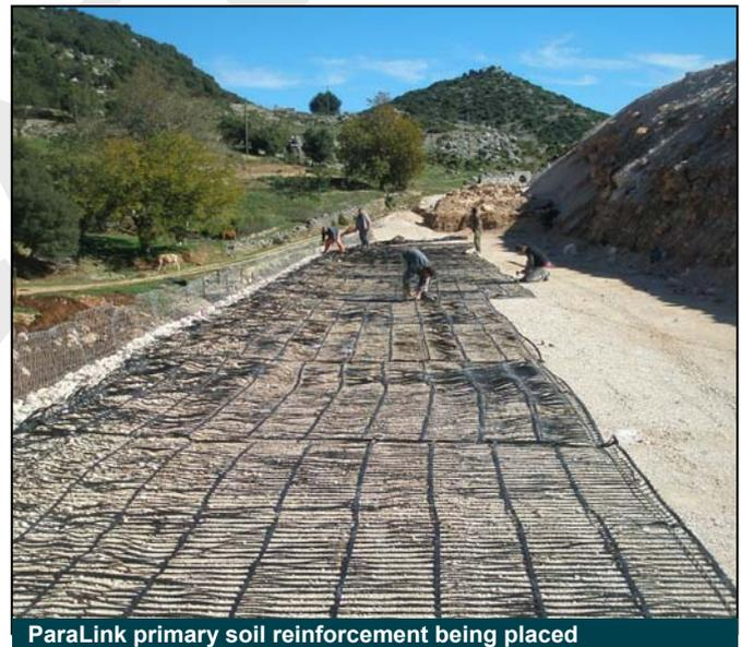
ParaLink primary soil reinforcement being placed
